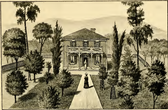
RESIDENCE OF GEO. S. GILBERT, SAN BUENAVENTURA, CAL.
